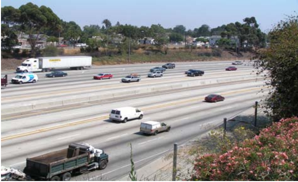
110 Harbor Freeway looking south from 120th Street
